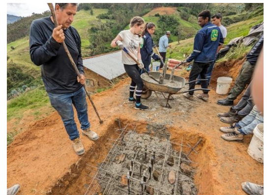
Figure 3- Mixing and working with the concrete on site
